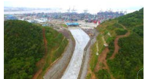
Ningbo Daxie planted vegetation on the slope of the road leading to the terminal
