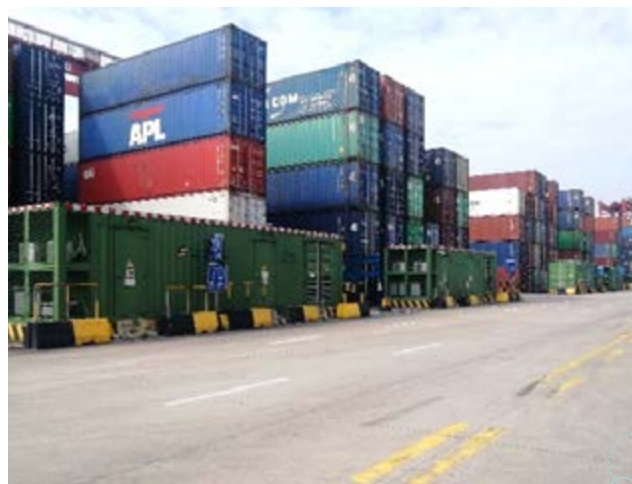
Shekou Container Terminal has completed the construction of 3 sets of shore-powered supply systems and it is expected to reduce emissions of 365 tons of carbon dioxide, 4.6 tons of sulphur dioxide, and 4.57 tons of nitrogen oxides by each berth annually.
